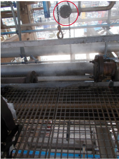
FIGURE 7. The location of the injection point discussed in Example 2 (highlighted by the red circle) challenges modification
