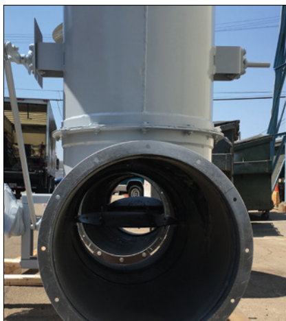
FIGURE 2. High-cycle butterfly valves used in RTOs will employ a flat valve plate that is mechanically rotated to control gas flow
